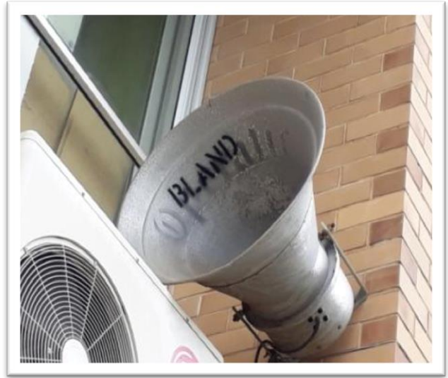
Bland Outdoor Horn Speaker using 8 Inch Speaker
